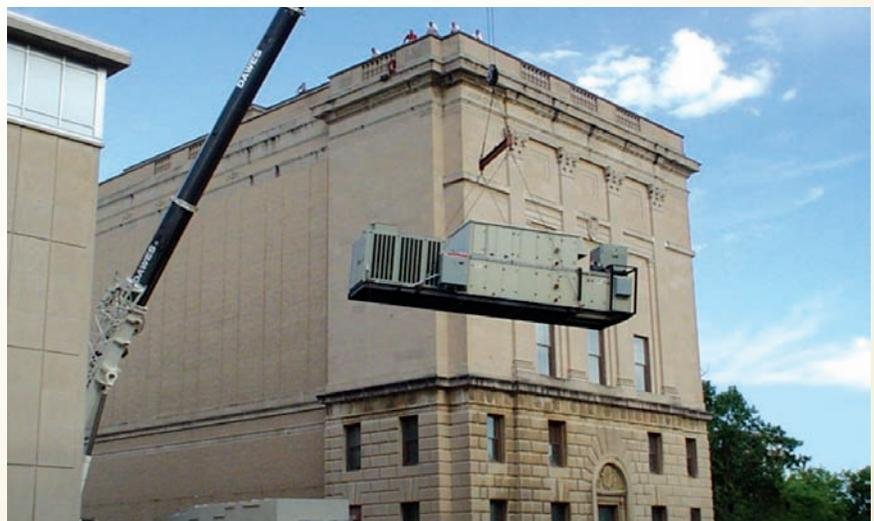
(Above) A crane removes the old dehumidification equipment from the building rooftop. (Top Right) A more efficient and effective Munters humidity control system was installed.
